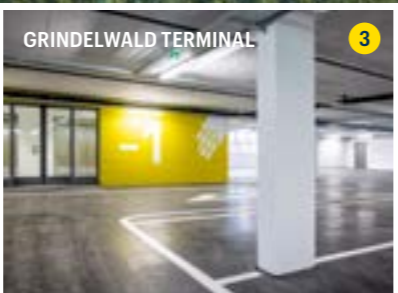
GRINDELWALD TERMINAL 3 Grindelwald Grund multi-storey car park
