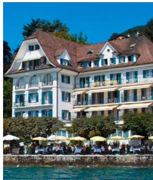
Hotel Central am See Weggis
