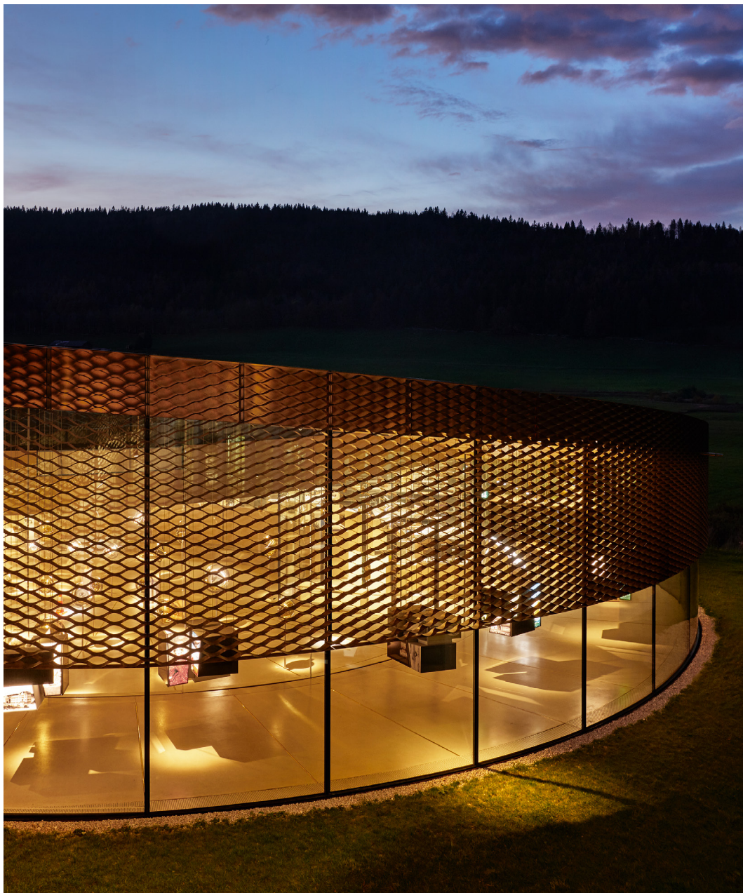
▲ The spiral designed by BIG is entirely supported by curved glass walls. A brass mesh runs along the exterior to regulate temperature and light, without obstructing the view.
